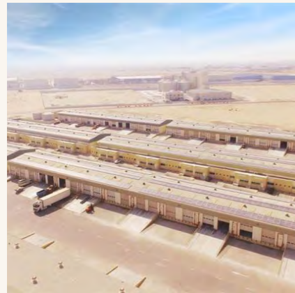
DP World Launches UAE's First Green Storage And Warehouse Facilities
